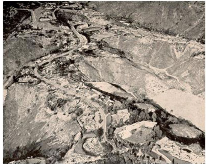
Figure 2. Ridge-top destruction after the Bel-Air Brentwood Fire. Source: LA Fire Department.
